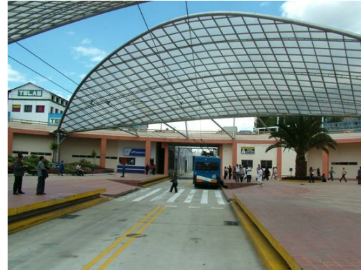
BRT transfer facility under grade-separated roundabout in Quito, Ecuador
