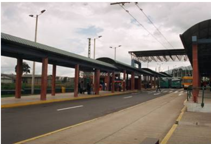
Transfer terminal between trunk and feeder lines, Quito
