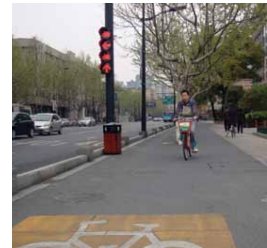
Clearly marked bike lanes and special bike stoplights improve safety for bicyclists.
