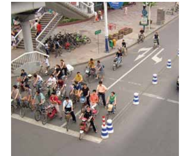
Bollards connected by wire help slow cars down as they turn right. Cyclists get a left turn arrow and have their own left turn lane in the protected bikeway.
