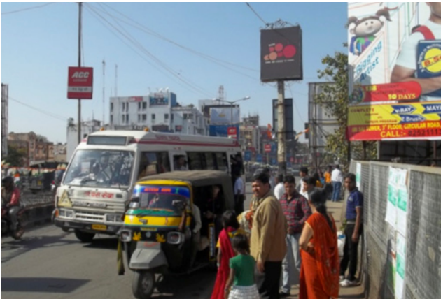
Most bus shelters are in poor condition (left) and at many stops there is no shelter at all (right).
