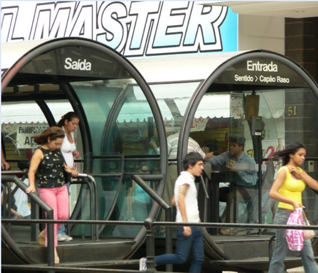
A bus rapid transit station in Curitiba, Brazil, takes passengers directly to the urban center.
