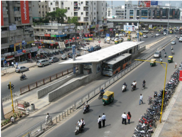
Figure 2.12 This BRT station facilitates high quality service for passengers since it is located in the median and operates with level boarding. It also leaves sufficient queuing space at the intersection.
