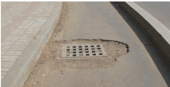
Figure 2.54 The joint between the drain cover and the surface of a cycle track is substandard and the placement of the drain in the cycle track means that cyclists ride through the deepest water in the cross section.
