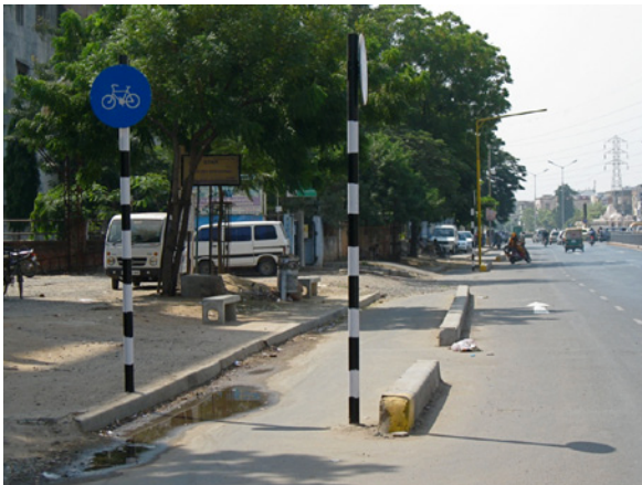
✗ Figure 2.7 This cycle track has four problems: (1) it is not continuous, (2) it collects water runoff and dirt because it is at the lowest point in the cross section, (3) it is not properly separated from the carriageway, and (4) the curbs and signpost reduce the usable width.
