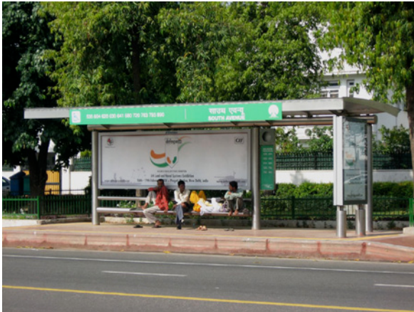
Figure 2.28 This bus stop provides protection from the elements, is elevated above the carriageway, displays customer information, and has a clear identity.
