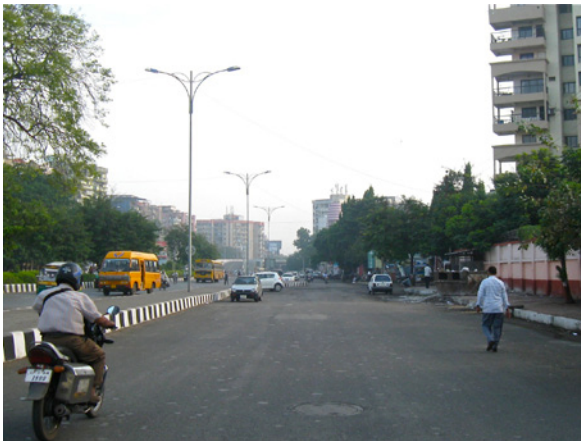
✗ Figure 2.45 This wide service lane does not function as a safe pedestrian space because it permits vehicles to travel at very high speeds.
