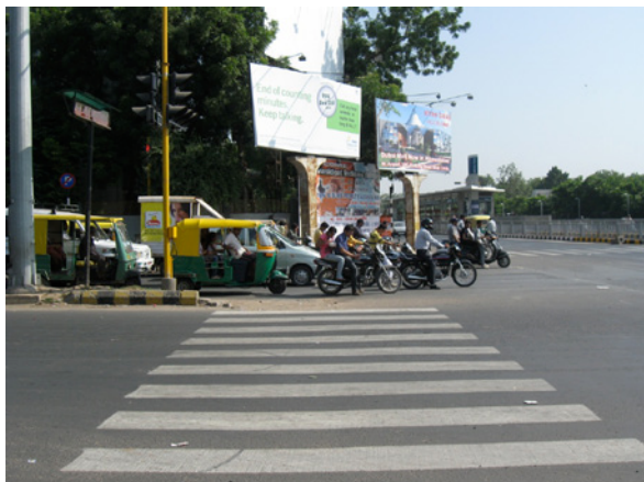
✗ Figure 2.22 This painted crossing is completely ineffective. Since drivers do not observe painted road markings, the only means of ensuring pedestrian safety is physical treatment, perhaps assisted by enforcement.
