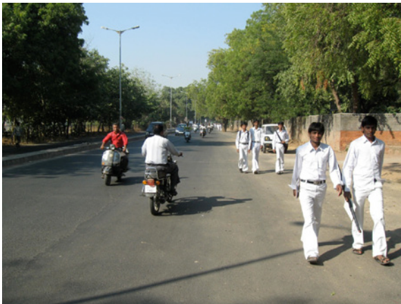
X Figure 2.10 The wall-to-wall carriageway on this street in an educational area sends a signal to pedestrians that they are not welcome. Also, the excessive width of the carriageway encourages speeding and wrong-way driving. Footpaths, cycle tracks, or markets would be a better use of this excess carriageway space.
