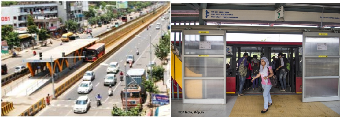
Figure 12. A BRT system provides high-quality and high-frequency mass transit system for the city. The system must have exclusive right-of-way for BRT buses, supported with high quality stations with IT based off-board fare collection system.
