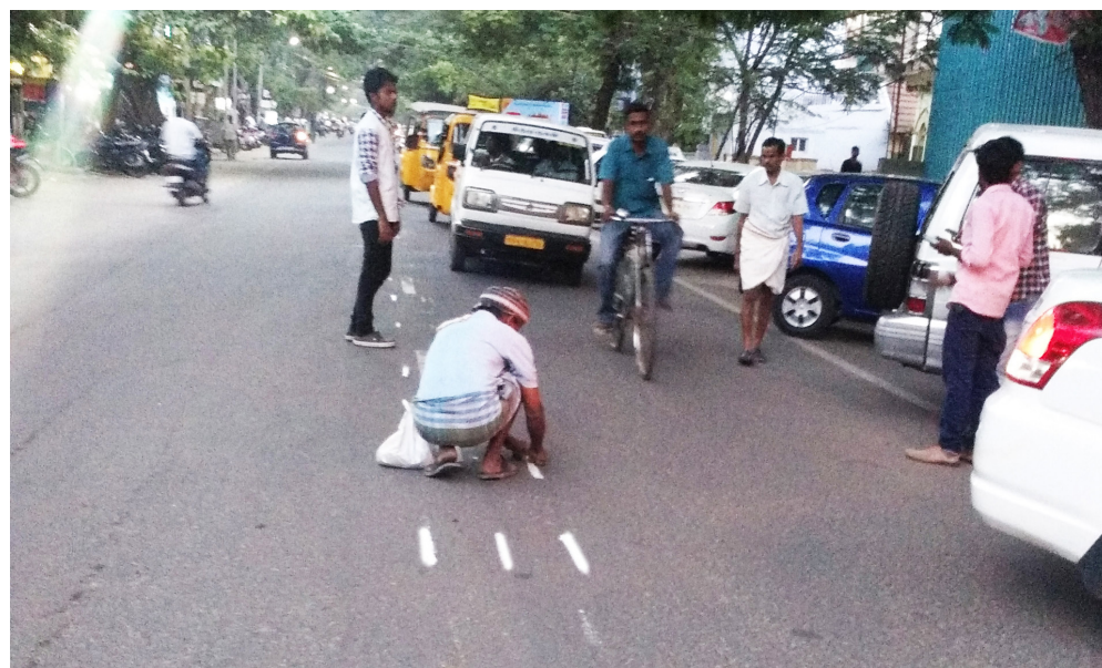
Fig. (above) Street centreline marking on a street in Chennai
