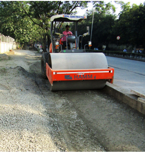
Fig. (top) Utility bed preparation and backfilling in FC Road, Pune Fig. (bottom left) Heavy roller for compacting surfaces without utilities beneath, as seen in University Road, Pune Fig. (bottom right) Walk-behind roller compactor in case of utilities underneath, as seen in FC Road, Pune
