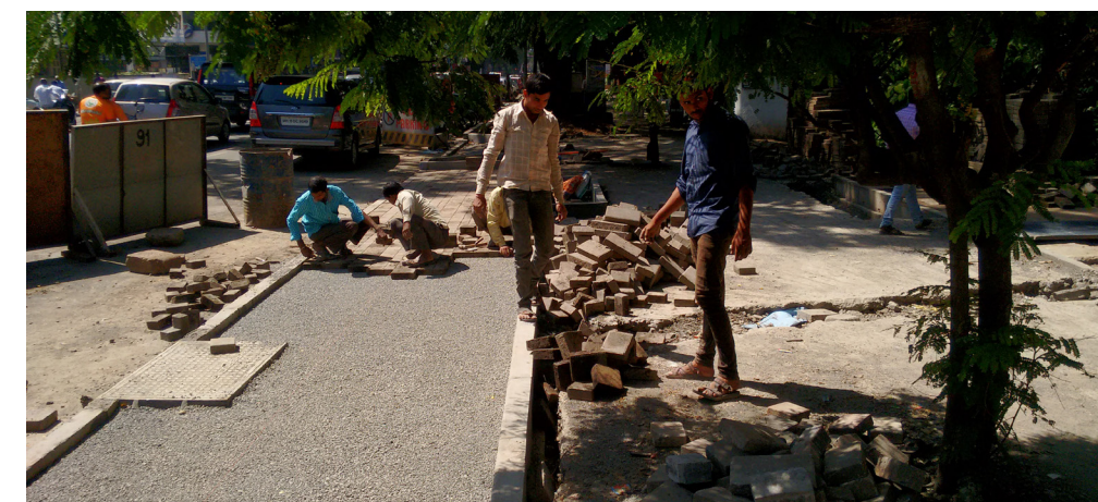
Fig. Paving tiles/blocks are laid on the compacted base to finish the footpath. This requires fine workmanship so as to ensure that the blocks are laid close together and do not come loose in the future.
