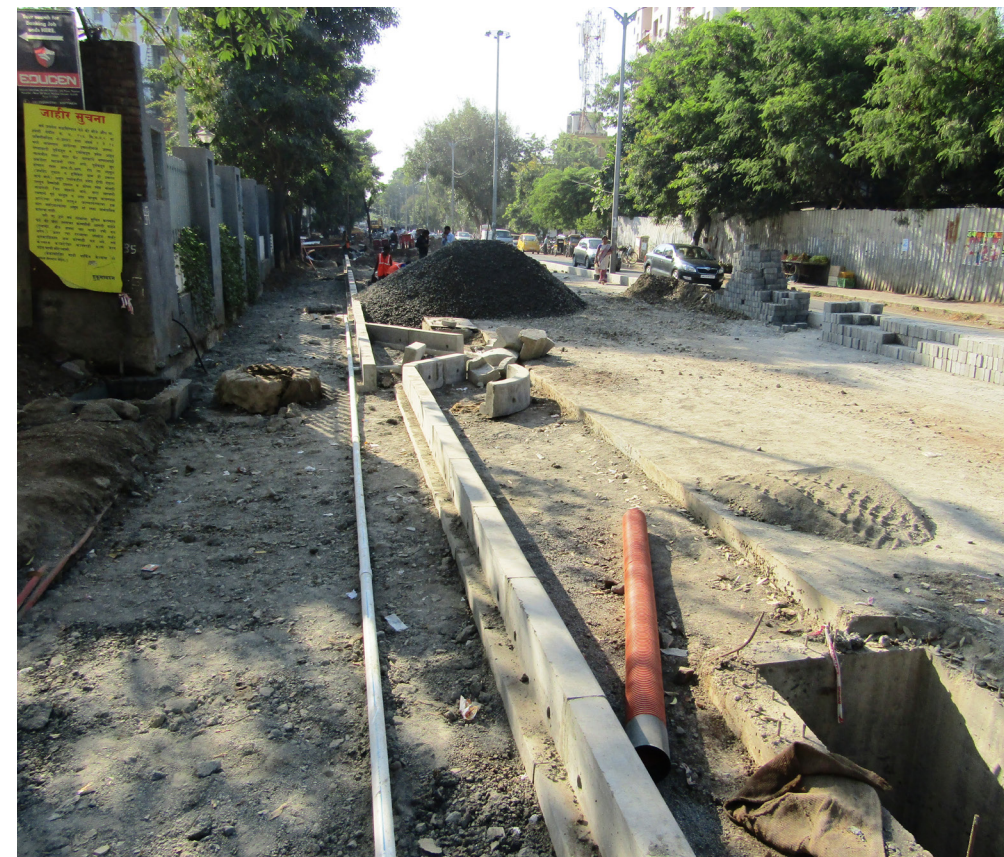
Fig. (above) Kerb stones are carefully placed over PCC mortar base maintaining the alignment and height in FC Road, Pune
