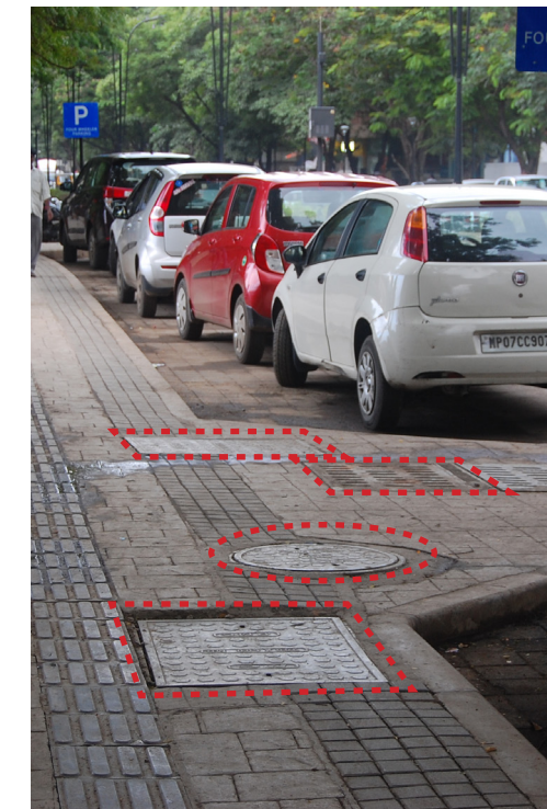
Fig. (top left) Manholes at bulbouts and utilities at tree pits in JM Road, Pune
