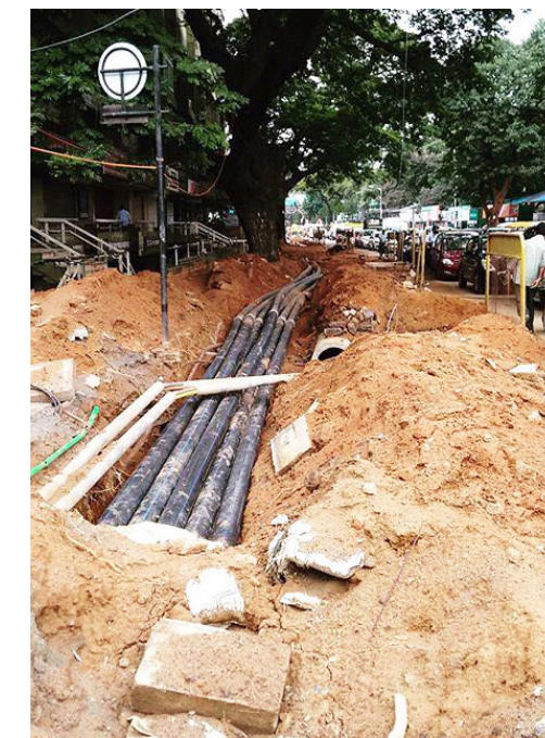
Fig. (left) Damage caused by excavating beyond 2m around trees in Coimbatore
