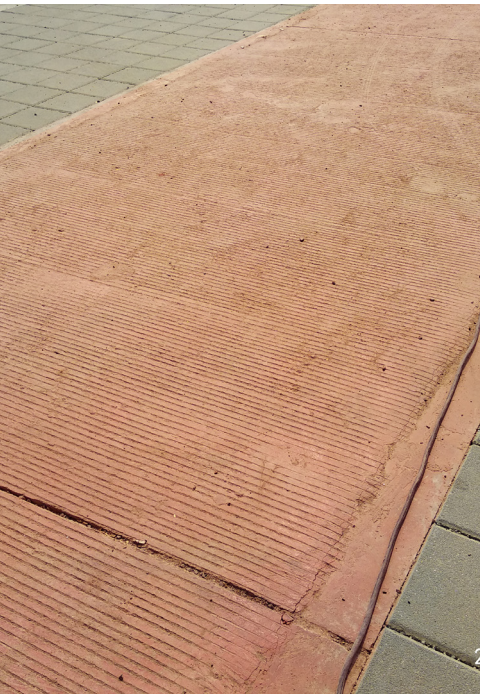
Fig. (top) Different surface finishes for different uses Fig. (bottom left) Broom finish for cycle tracks in FC Road, Pune Fig. (bottom right) Broom finished pigmented surface for cycle track
