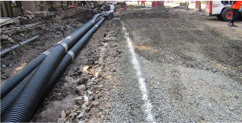
Fig. (top left) Workers manually levelling the granular sub-base in DP Road, Pune Fig. (top right) Sub-base under construction in JM Road, Pune Fig. Alignment lines are drawn to mark the kerb, cycle track, pedestrian and green zones
