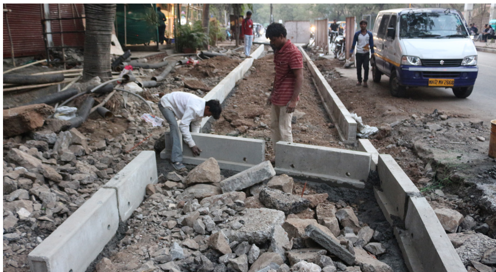
Fig. (above) Alignment of kerb stones as per design in JM Road, Pune
