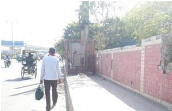
Image 6: Utilities impeding the pedestrian movement
