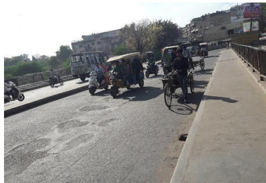
Image 11: Absence of street light around Okhla bus terminal
