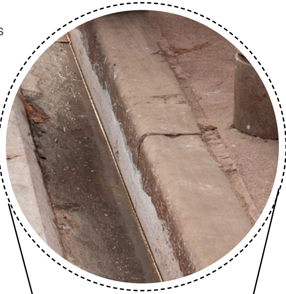
Precast Concrete Drainage Channels installed along the street edge.
