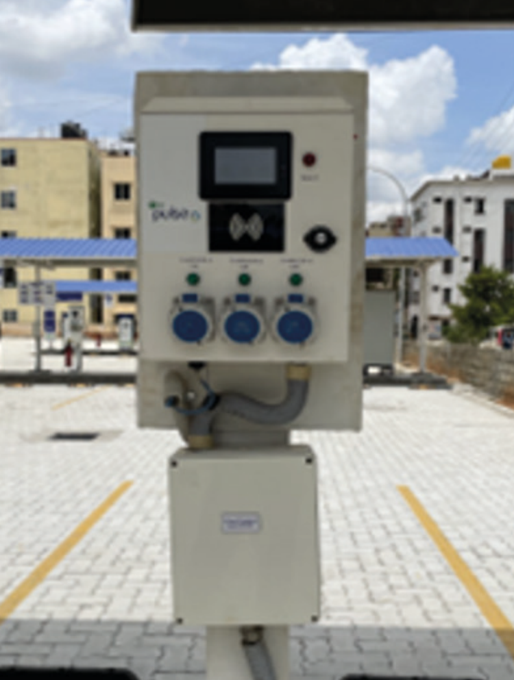
Figure 20,21 & 22: EV Charging stations(7.5 kw, 30kw, and 60 kw) (Photo: ITDP)
