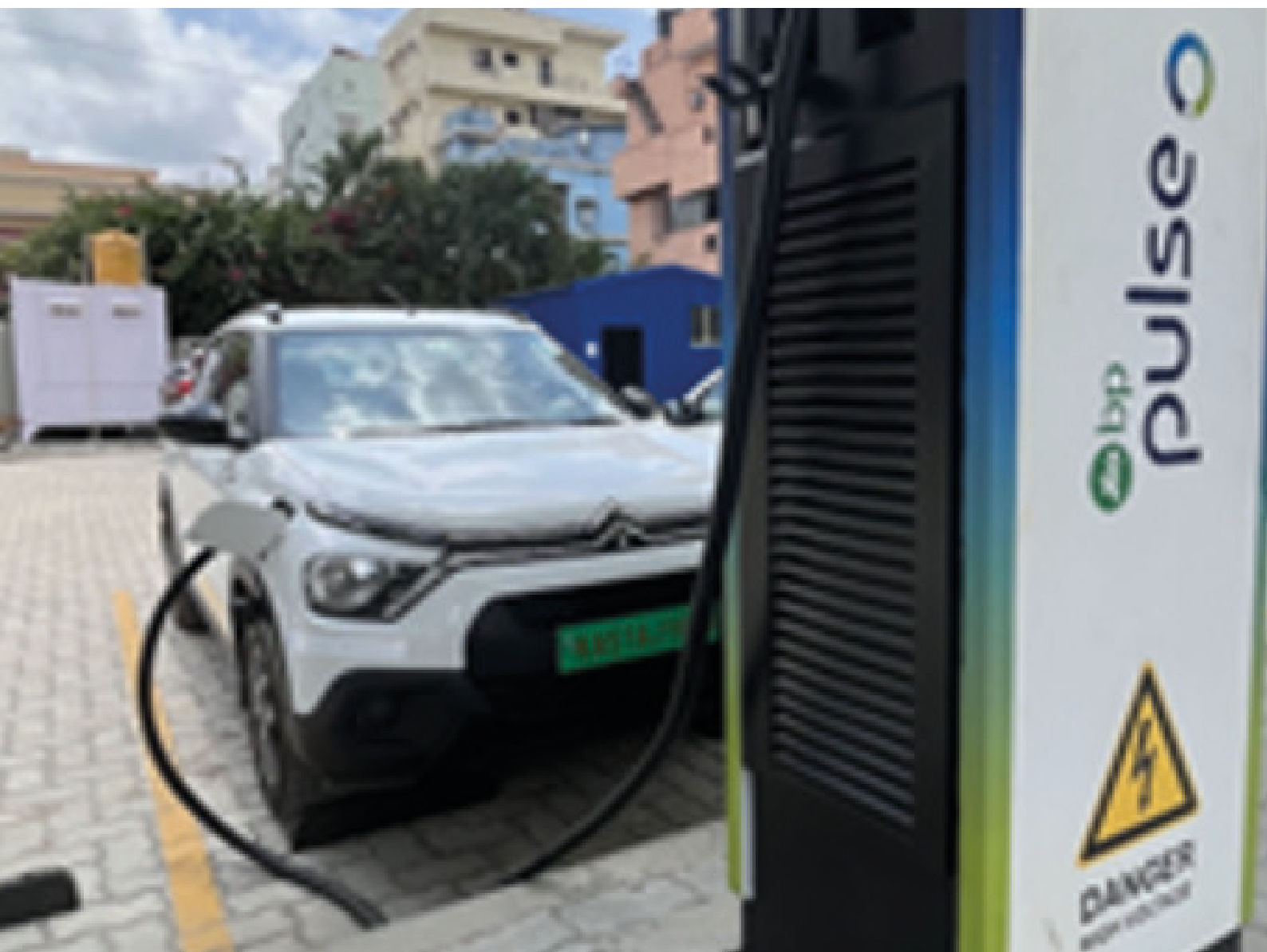
Figure 20,21 & 22: EV Charging stations(7.5 kw, 30kw, and 60 kw) (Photo: ITDP)
