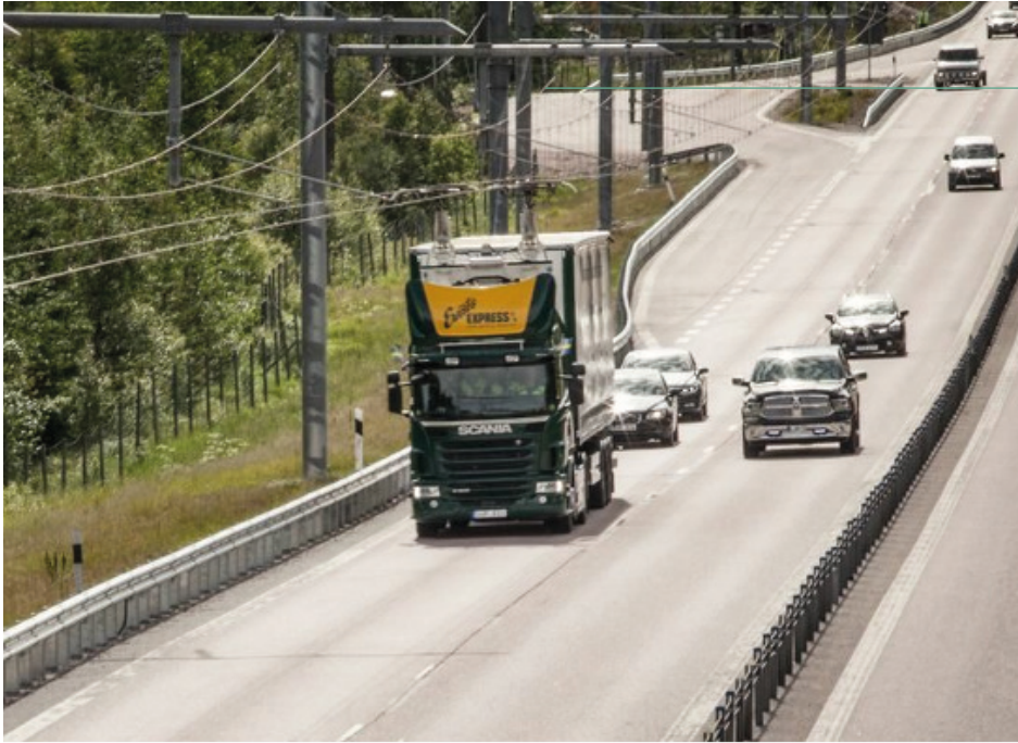
Figure 9: E-highways in Germany established by Siemens 22
