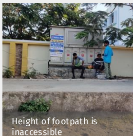
Stormwater drain finished as footpath
