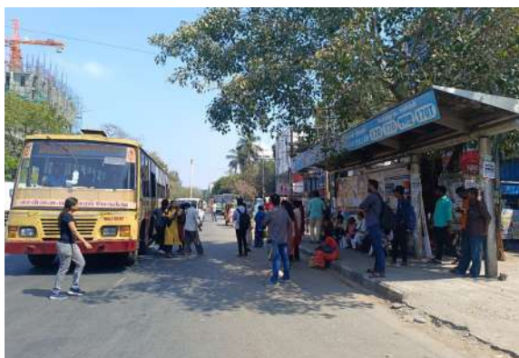
Stand-alone bus shelter
